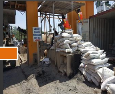
Pengolahan hotmix aspal karet di Asphalt Mixing Plant (AMP)
